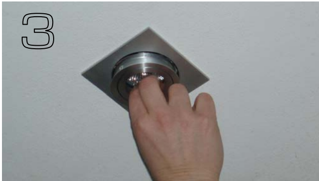
3 Remove by pulling eyeball assembly straight out
