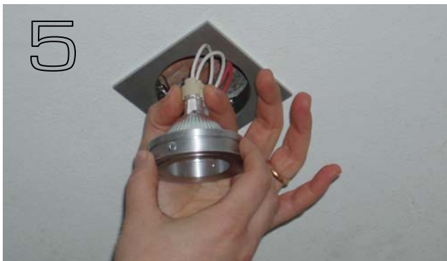
5 Separate lamp from socket, being careful not to put stress on lead wires.
