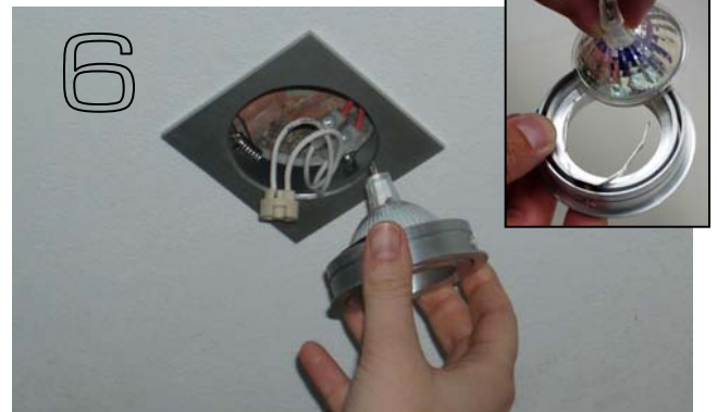
6 Release lamp from retaining clip. Replace with new lamp and reverse procedure.
