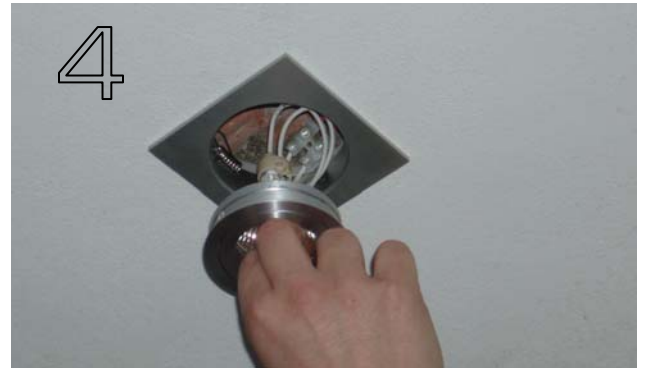
4 Lamp and socket are now accessible
