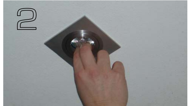
2 Grasp inside wall of eyeball assembly
