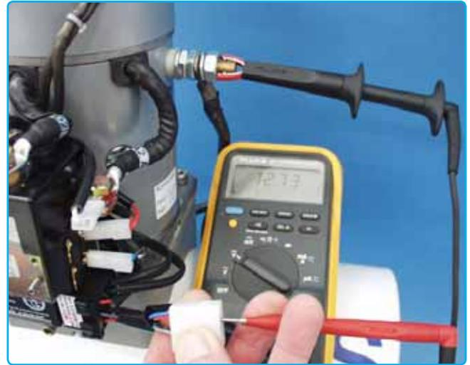
*Checking voltage on motor harness to battery negative stud*
